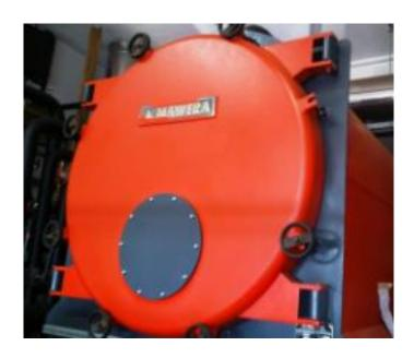
Long before it was popular to do so, DW Mouldings have been burning their waste sawdust and chippings to produce heat for their 3084m2 factory. With the inclusion of a finishing line in 1999, the heat from the boiler was also used to dry their finished products.
