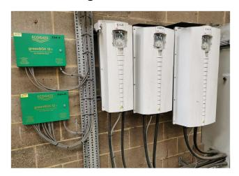
The Green Box was installed on our extraction system and it soon proved to have more advantages than we anticipated. By directing suction exactly where it's needed in real-time using intelligent controls, Ecogate systems use one-third the electricity of those traditional systems while making every other part of the system work better. Air quality, electricity use and noise levels are all improved.
