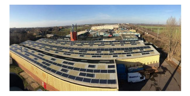
DW Mouldings continue their commitment to the environment, with the installation of 460no high performance 'Winaico' photovoltaic modules. With an estimated annual output of 106,605 kWh, it has reduced our demand for electricity from outside sources.
